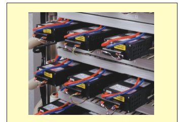
CMR panel door showing the rear of the DPMs. Designed for easy access during calibration in future.
